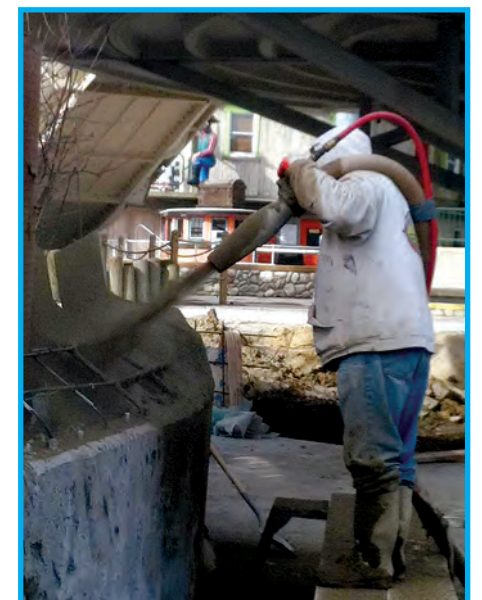
A worker Shotcretes the new river at Raging Waters.
