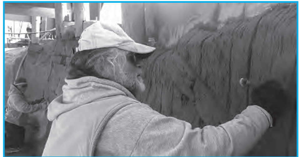
Steve Pez, "The Steak Knife Wielder", seen here sculpting the freshly poured concrete to look like distressed wood with his signature tool.
