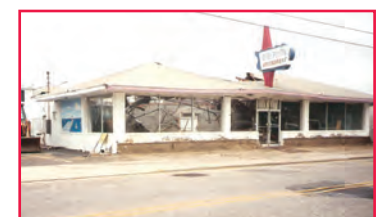
Demolition of the Dolphin, 2002
