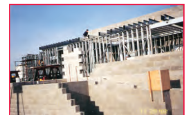
Construction of Star Diner, 2003
