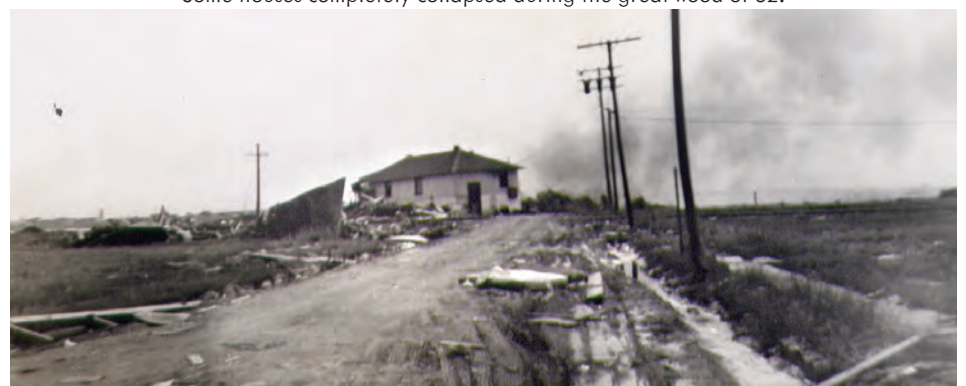
Devastation can be evidenced in this photo of debris and eroded streets, taken near Otten's Harbor
