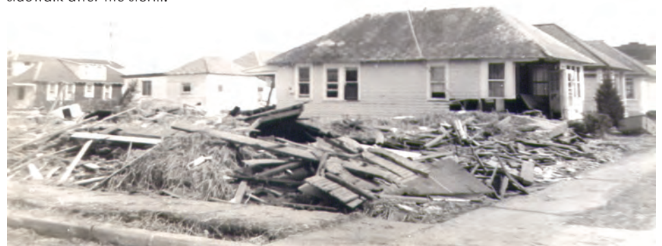
Some houses completely collapsed during the great flood of 62.
