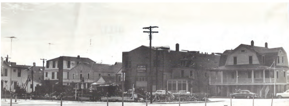
The ruins of Nesbitt's Furniture Store, looking at Schellenger Ave.
