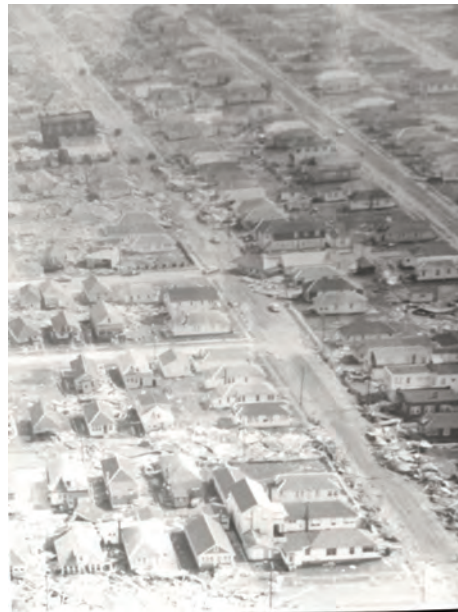
Aerial view of the storm damage over West Wildwood
