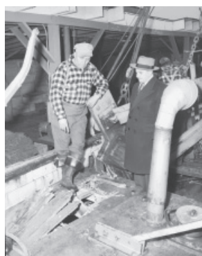
Capt. Friesenborg with insurance company photographer assessing the damage to the Irma Pauline after the George Redding bridge went down on the masts.
