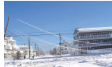
sagging wires on Ocean Ave., NWW
